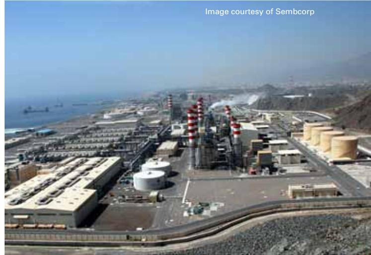
Fujairah Independent Water and Power Plant (IWPP), UAE – As the world's largest operating hybrid desalination plant, the Fujairah IWPP has a desalination capacity of 100 million imperial gallons of water per day.
